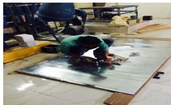
Fig. 4. Fixing Of Thin metal Sheet On Plywood
