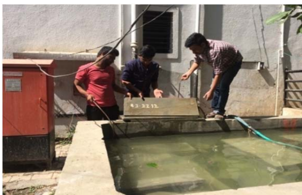
Fig. 7. Curing of Panels
